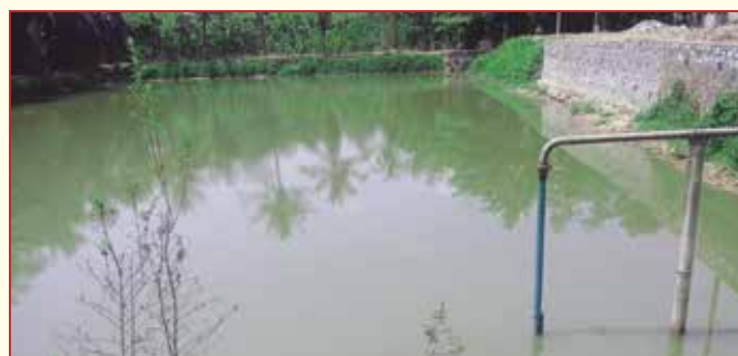
Water tank for water harvesting for rain water
